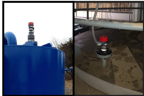
Tracer 2G with 1½" NPT mounting in liquids, slurries or solids applications.
