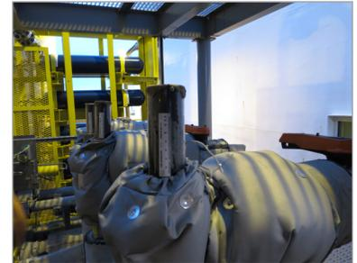
Figure 4. FLO-CORP's MEMFlo™ MFVC Volumetric (VA) Flow Meter installed on a compressed air system.
