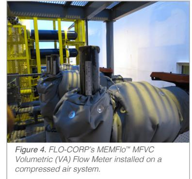
Figure 4. FLO-CORP's MEMFlo™ MFVC Volumetric (VA) Flow Meter installed on a compressed air system.
