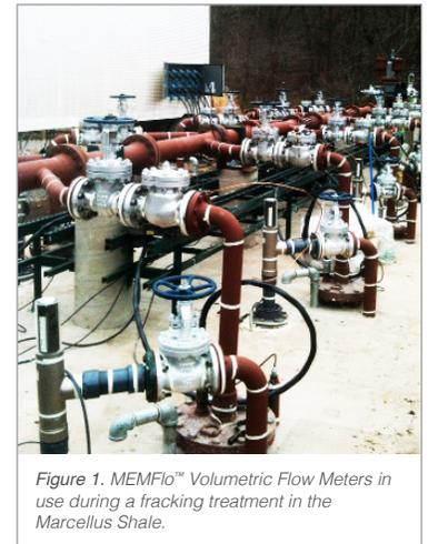
*Figure 1. MEMFlo™ Volumetric Flow Meters in use during a fracking treatment in the Marcellus Shale.*
