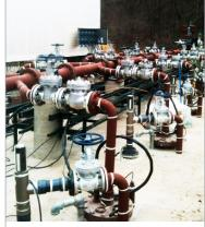
Figure 1. MEMFlo<sup>™</sup> Volumetric Flow Meters in use during a fracking treatment in the Marcellus Shale.
