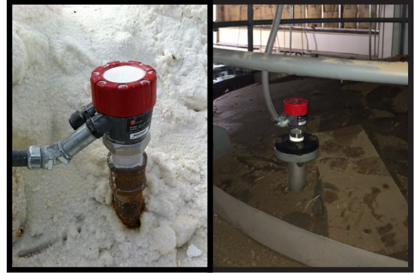
Tracer 2G with 1" NPT mounting in liquids, slurries or solids applications.
